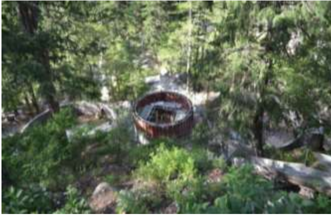
Sewage Treatment Plant At Gangotri
