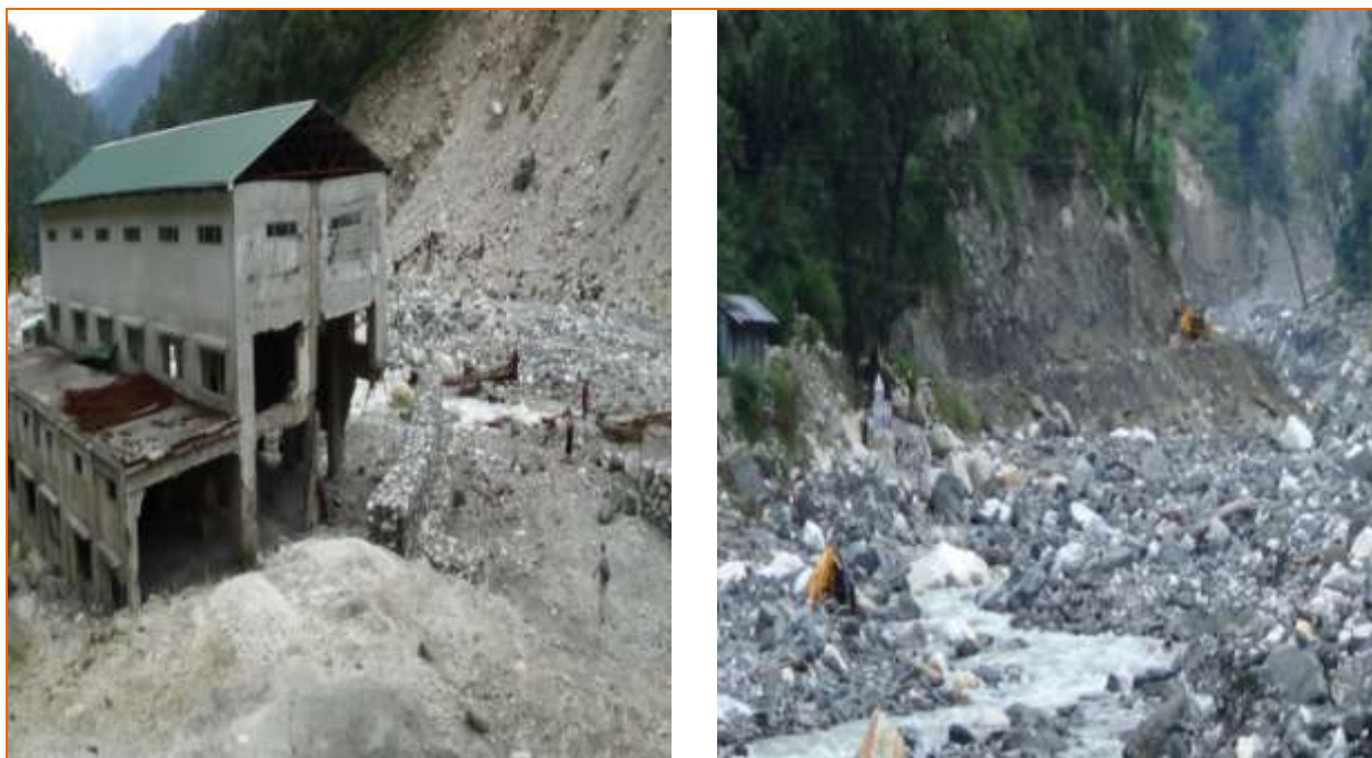
Pics. 37 and 38. Damaged Asi Ganga I Hydroelectric Project Site
