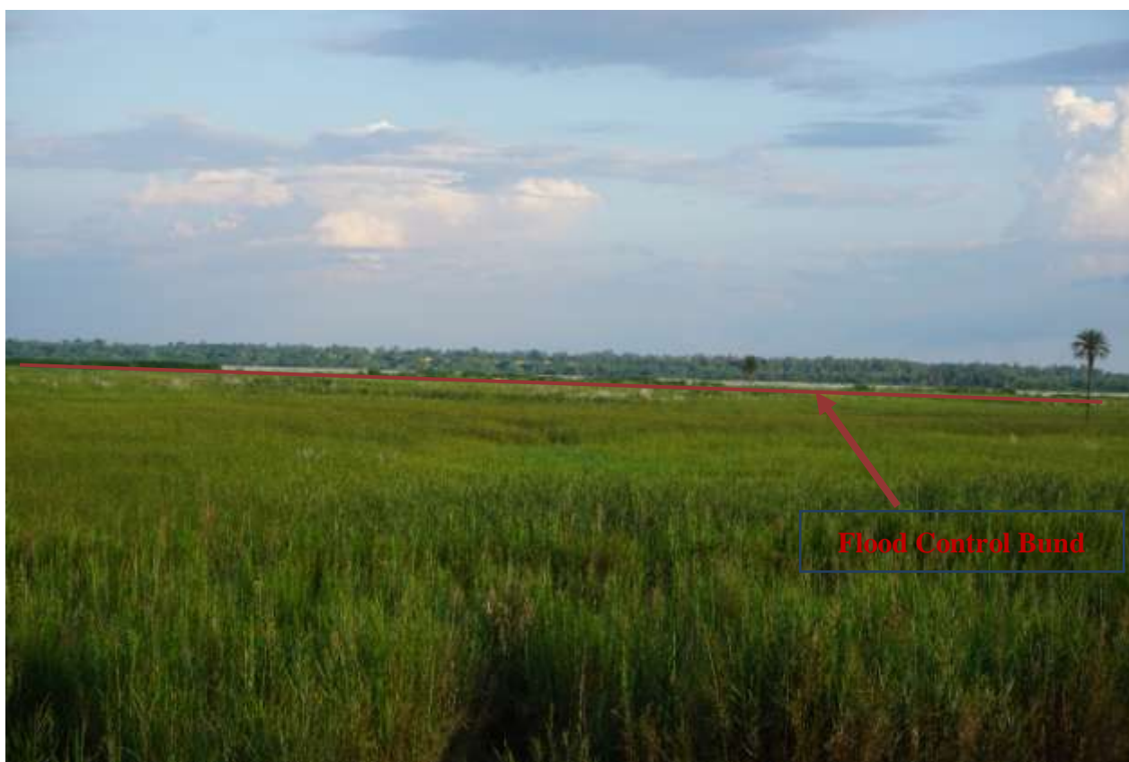
Pic. 185 : Shivpuri Wetland and Flood Control Bund
