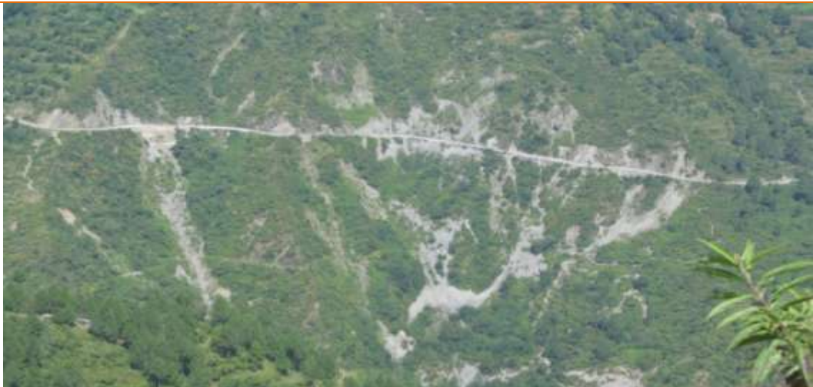
Pic. 42. Unstable upper and lower slopes after road constructions
