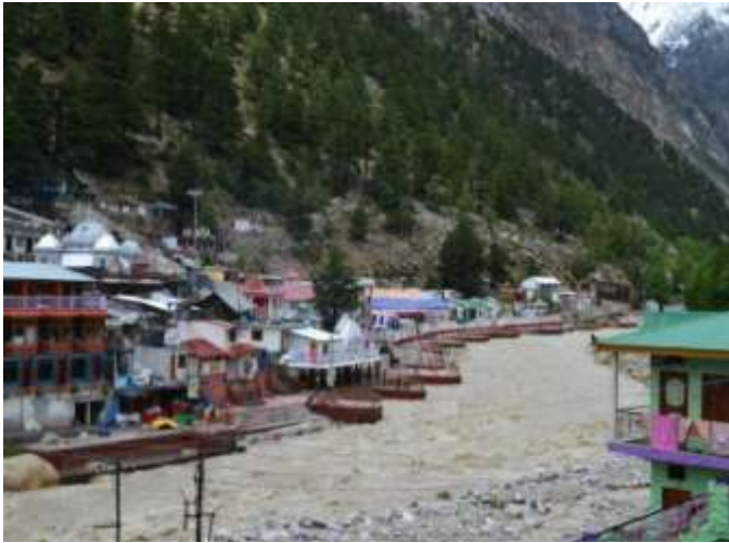
Unmonitored Construction In Gangotri Town
