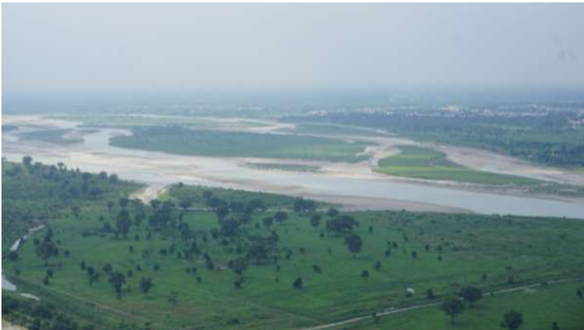
Pic. 127 : View From Hilltop Showing Active Floodplain Of Ganga In Haridwar City
