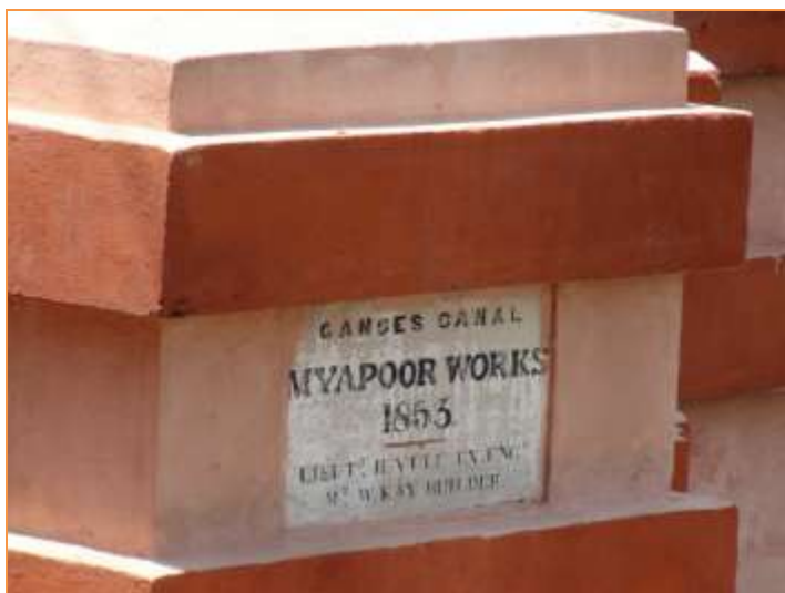
Pic. 94. Foundation Stone of Upper Ganga Canal
